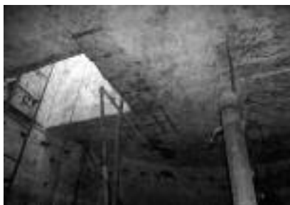
Strop obiektu The ceiling of the facility
