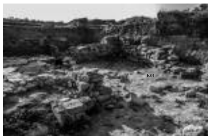
Fot. 2. Mury dzikie w Tyritake [Fot. E. Skóra] Photo 2. Irregular stone masonry walls in Tyritake
