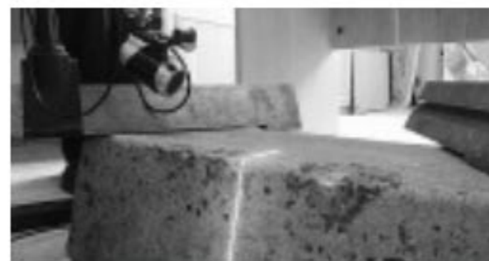
Photo 1. Scanning the surface of reinforced concrete sleeper
