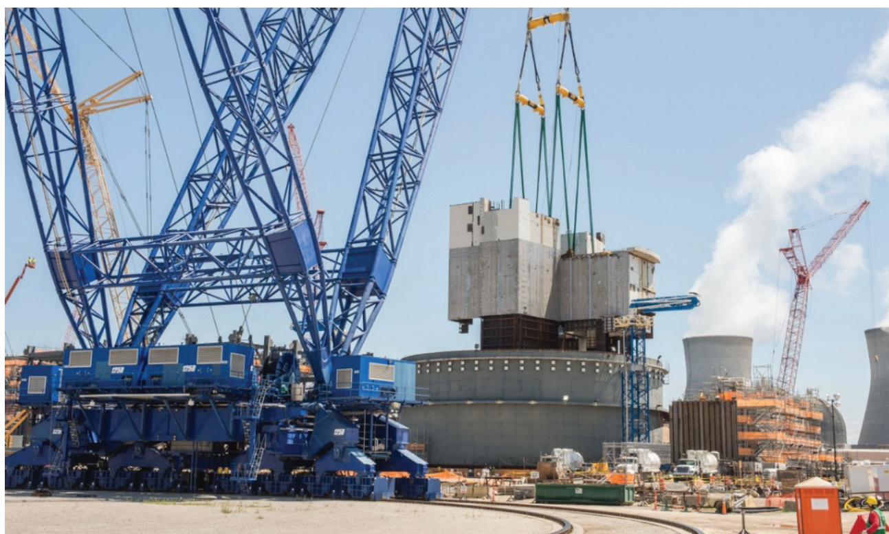
Photo 3. Structural module CA01 during installation into the containment vessel
