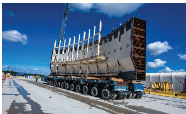
Photo 2. Shield building panels during transport on the construction site
