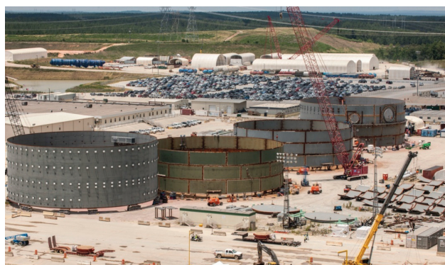
Photo 1. Containment vessel rings during erection
