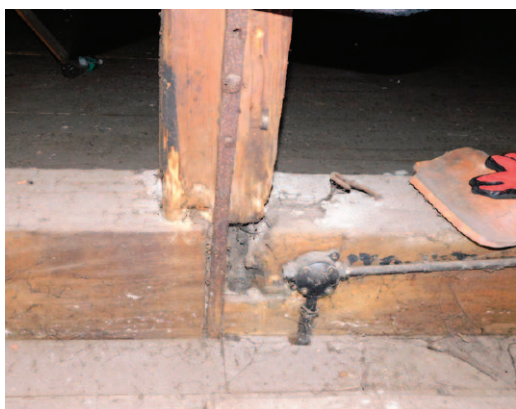
Photo 2. Old feeding site of larvae of the old house borer located in the lower part of the king post
