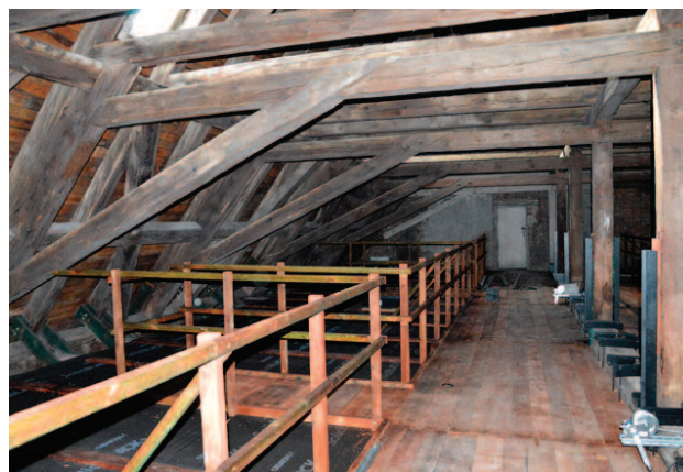
Photo 10. Lower part of the roof structure after strengthening
