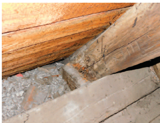
Photo 3. Old feeding site located in the lower part of the rafter with a visible carpenter's mark
