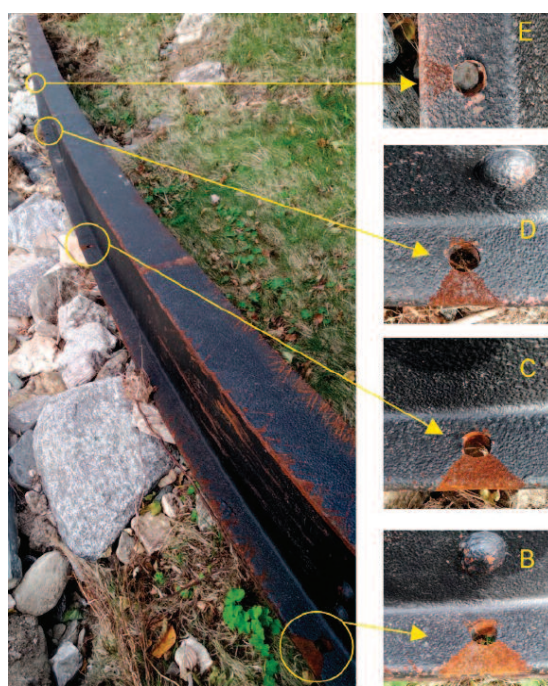
Photo 4. The range of plastic zones at the openings going from cross-section B (span) to cross-section E (at the support)
