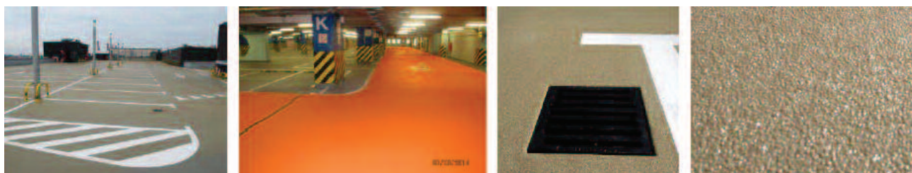
Photo 3. Polyurea parking surface made using Overspray technology [1]
