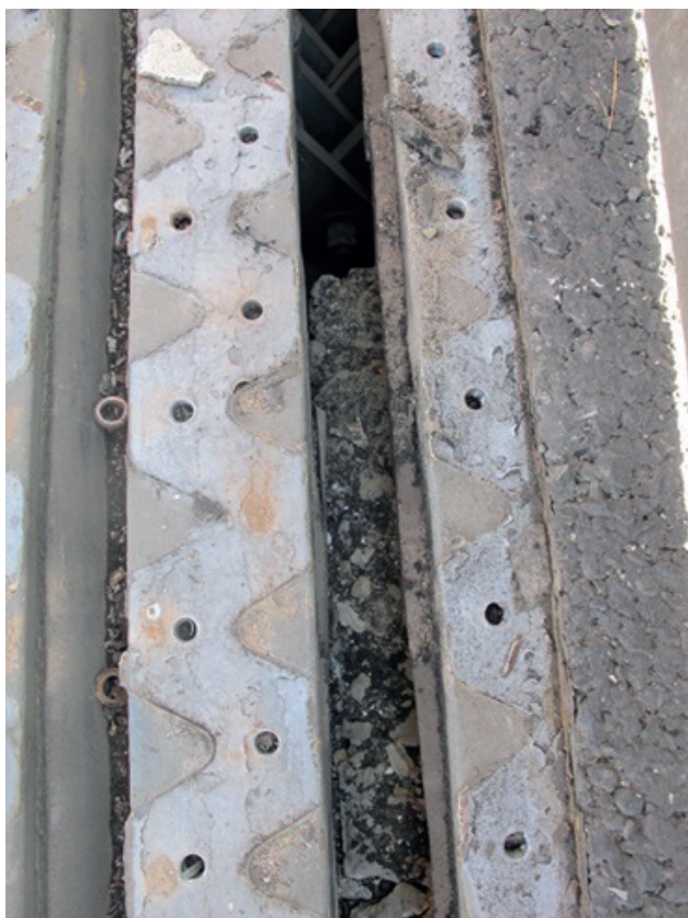
Photo 4. View of the hardened concrete mixture between the profiles of the modular expansion joint
