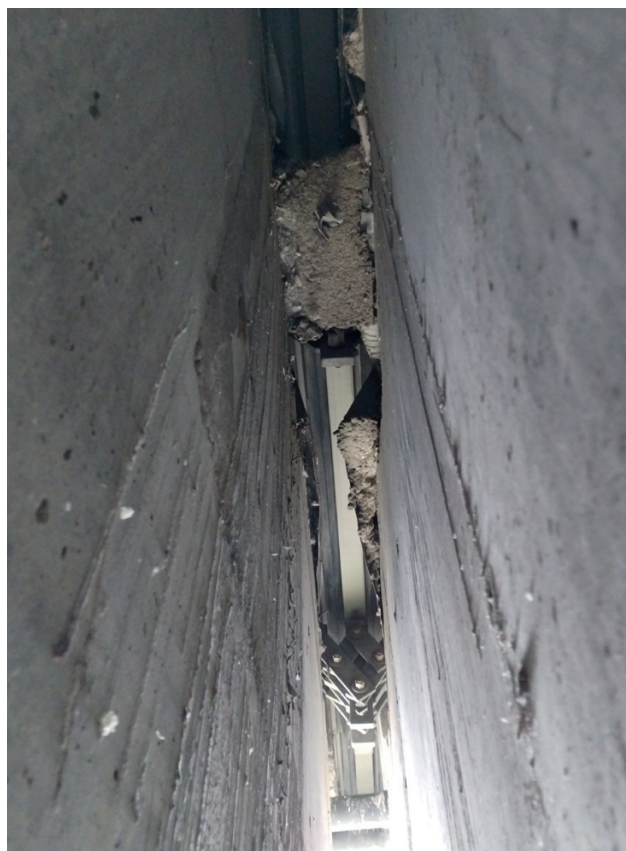
Photo 5. View of the hardened concrete mixture filling the expansion joint gap
