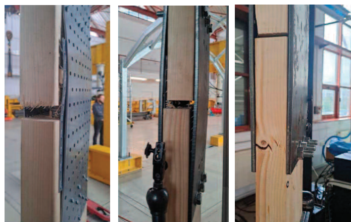
Photo 3. Failure of GR3 group joints: a) PKPG, PKBS; b) PKBS – transverse wood cracking
