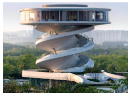
Photo 4. Observation tower in Nanchang (China) [7] Fot. 4. Wieża widokowa w Nanchang (Chiny) [7]
