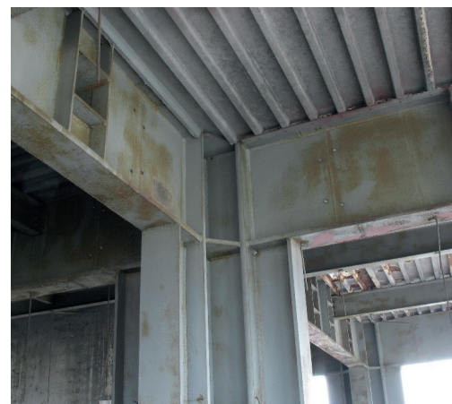
Photo 2. Steel frame junction (the decoupled communication core is visible in the background)
