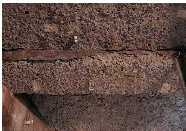
Photo 1. Concrete corrosion
