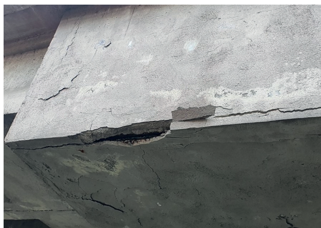
Photo 2. Frost-caused damage
