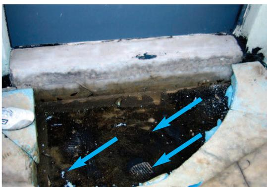
**View of the of the polymer-modified asphalt thick coating at the threshold of the door leading to the terrace, with traces of local thickness reduction. The arrows show examples of areas of coating thickness reduction in the region of increased local, pressure**
