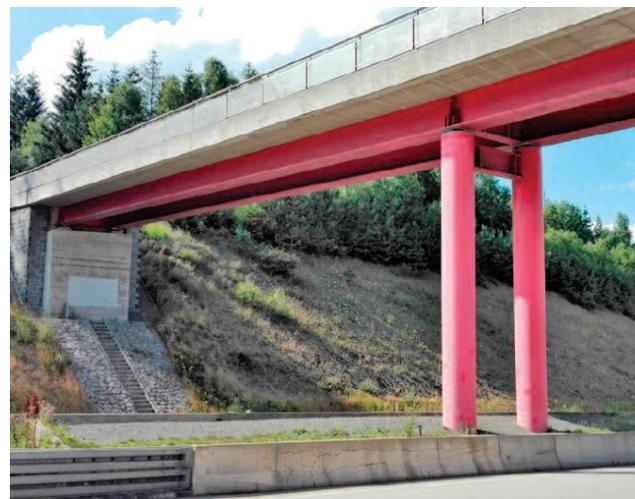
**An example of CFST columns application: composite steel and concrete bridge over the A93 highway between Hof and Regensburg in Germany**
