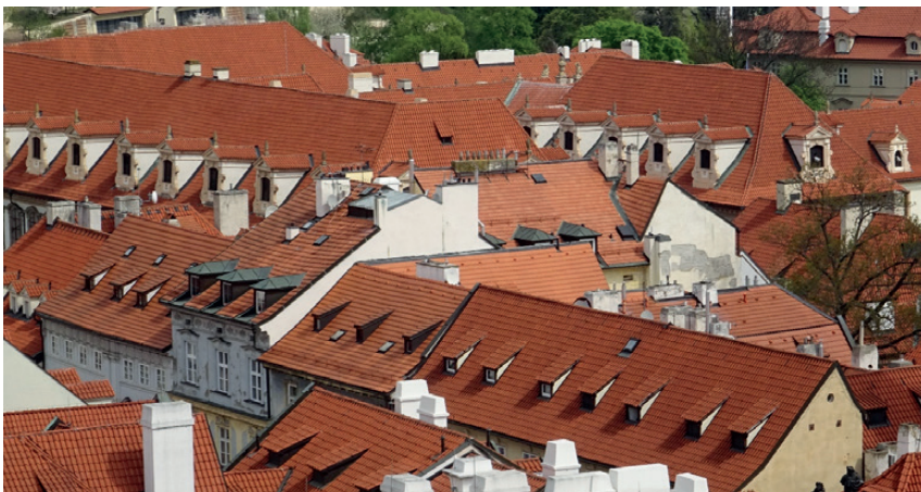
Fot. 1. Pokrycia dachowe – Praga, Czechy Photo 1. Roof coverings – Prague, Czech Republic
