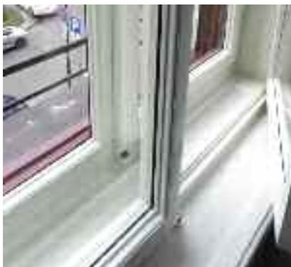
**Photo 3. Window in the historic building – a state after thermorenovation – window frame with glass panel (Type 2)**
