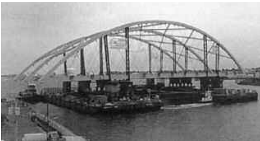
Fot. 5. Rhode Islands Providence River Bridge podczas transportu wodnego [Federal Highway Administration, Lifting the Graves Avenue Bridge to Success . Washington, DC. 2006]
