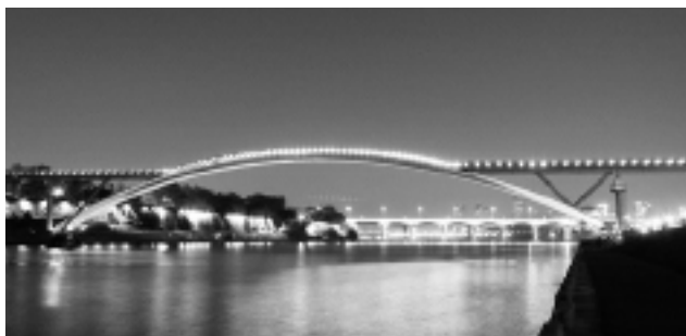
Most dla pieszych w Sunyudo [3] Sunyudo Footbridge [3]
