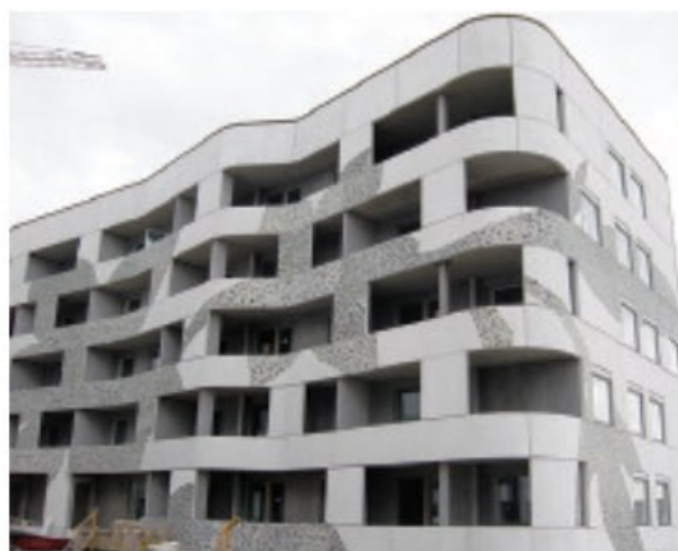
Fig. 10. Residential building with precast insulated sandwich panels
