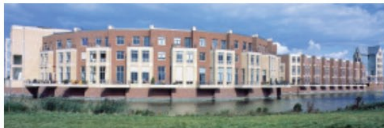
Fig. 7. A residential project in the Netherlands. The shape, layout and colour of the project illustrate the versatility of precast concrete and its adaptability to the requirements of the builder and the architect
