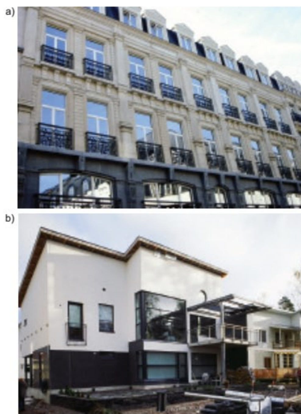
Fig. 8. The restoration of a traditional, classical natural-stone-masonry façade with architectural concrete elements in Brussels (a). There is no visual difference between the new façade in precast concrete and the traditional neighbouring façades; A precast single-family house in Finland (b)
