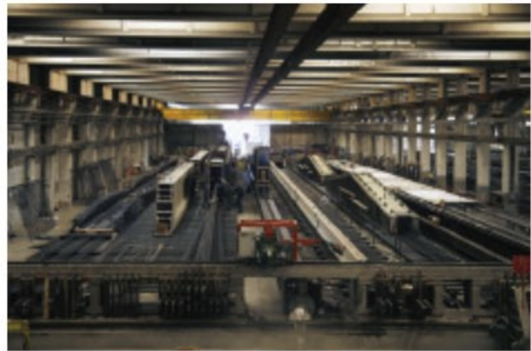
Fig. 5. Prestressing methods use long-line casting beds of between 100 – 180 metres in length
