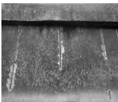
Photo 4. Corrosion of reinforcement Fot. 4. Korozja zbrojenia
