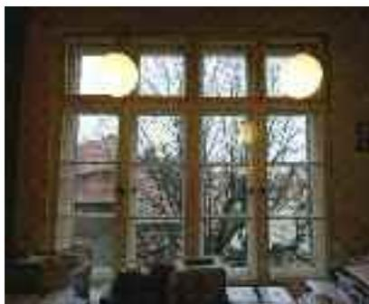
**Photo 2. A window in a historic building (Type 1) – a state before thermorenovation**
